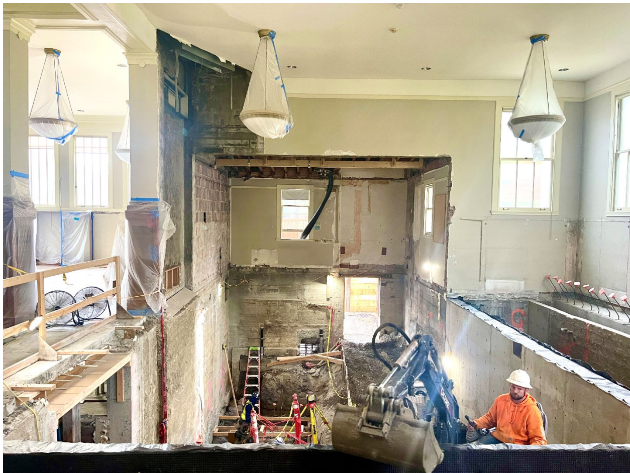
Green Lake Branch seismic retrofit work
